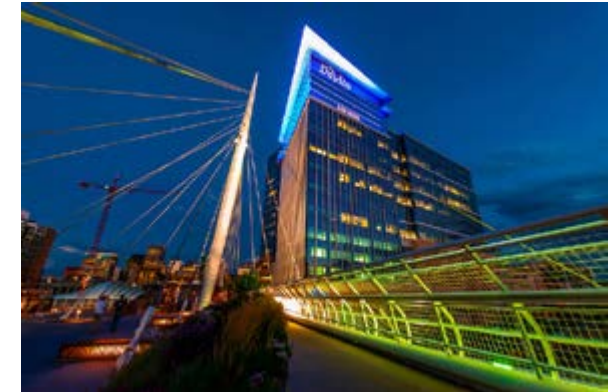
▲ Denver Millennium Bridge - Image by Blaine Harrington III
